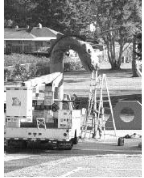
City workers install the repaired Dragon.
